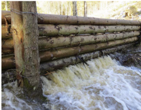
Central part of one of the two experimental timber bunds in the River Seven catchment
