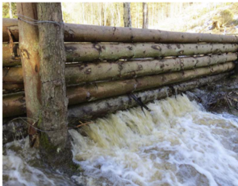
Central part of one of the two experimental timber bunds in the River Seven catchment
